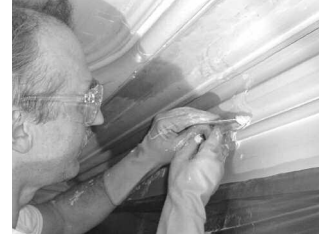
Restoration expert Rory Brennan repairs Dining Room moulding.
